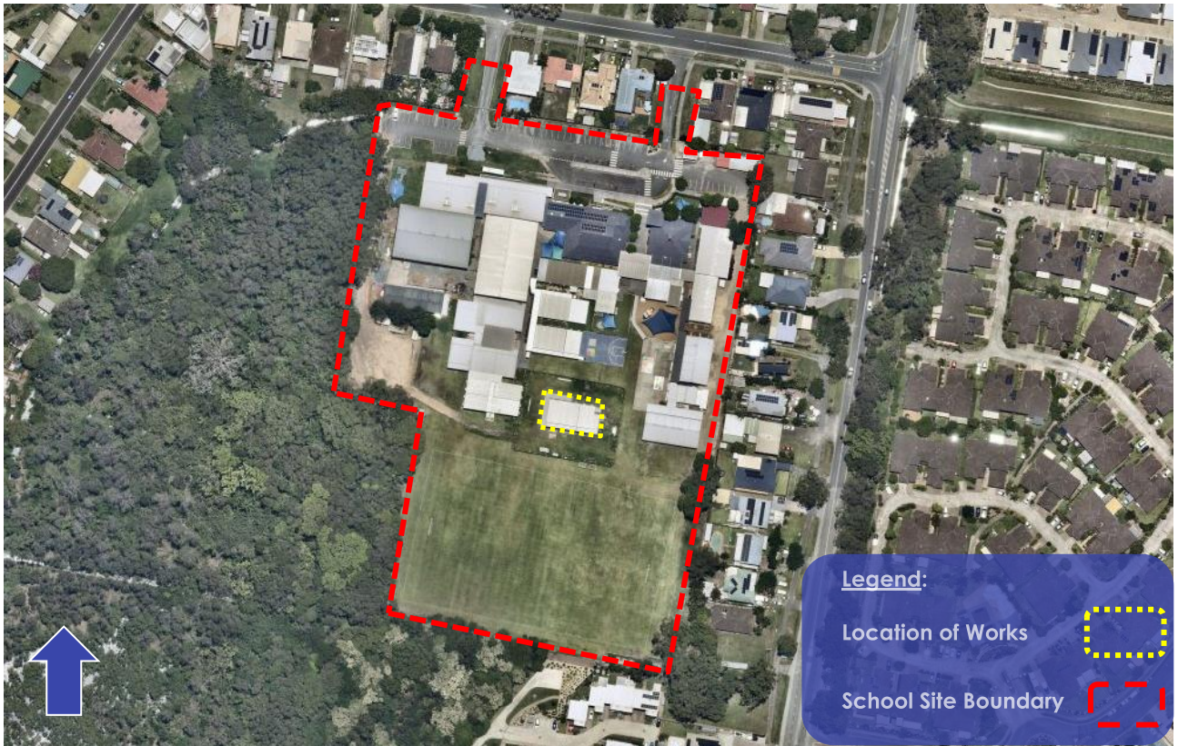
Figure 1: Aerial photograph of site indicating location of proposed works (in yellow) (source: Nearmap, dated 28 December 2023).
